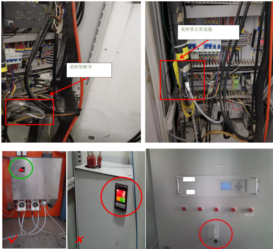
进样管路被人为钻孔示例图，进样管路接三通被稀释示例图
